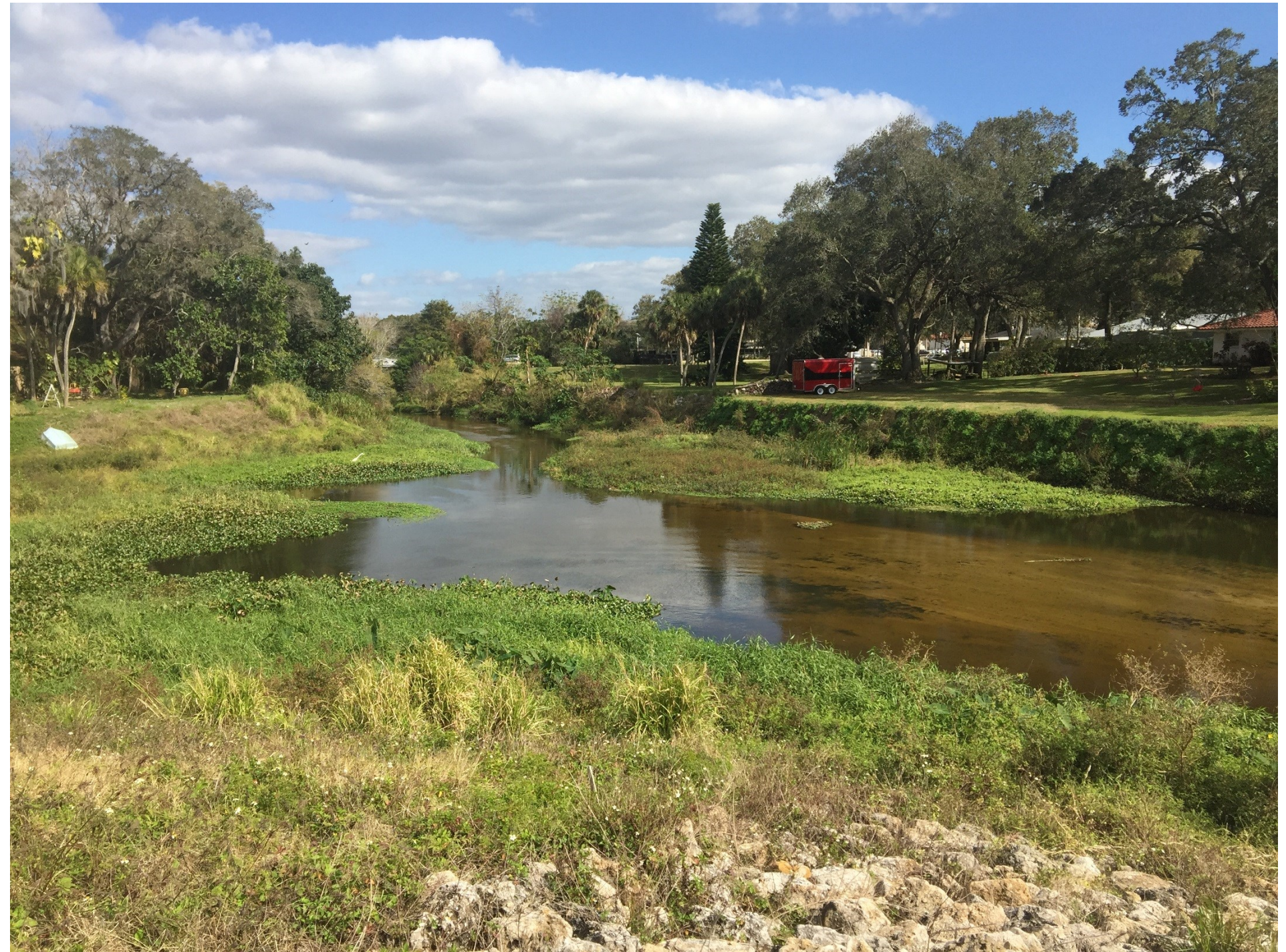
Sediment management system in the Phillippi canal network. Rocks in foreground are the staging area for cleanout equipment during routine maintenance dredging activities.
