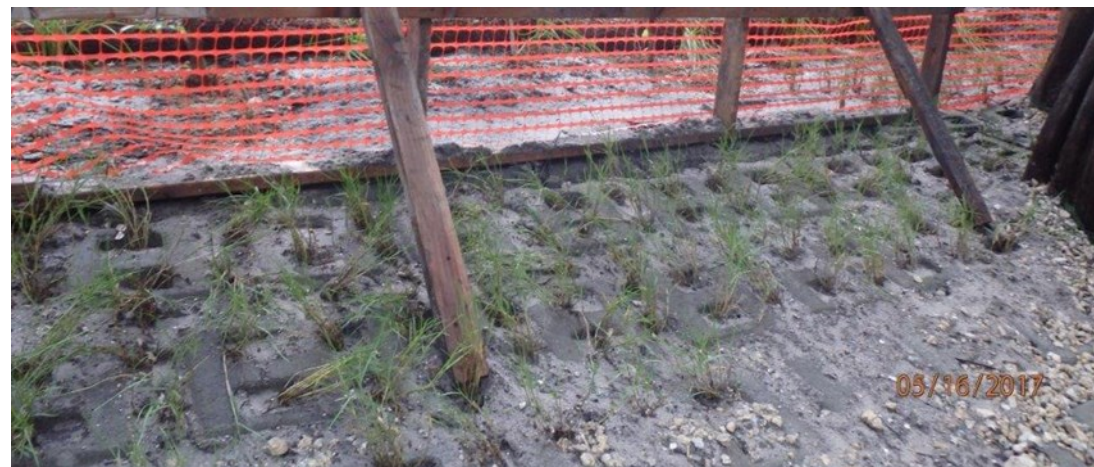
Open cell articulated concrete block, Loxahatchee River Florida.
