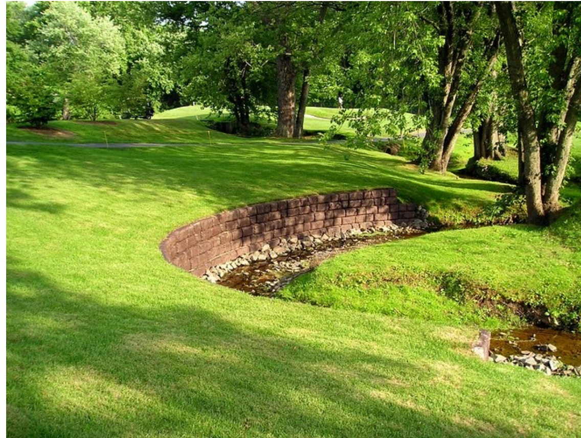
Textured segmental block concrete retaining wall.
