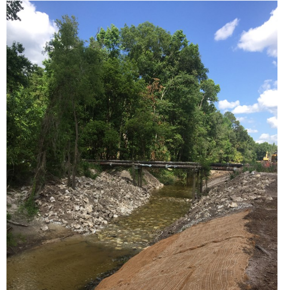
Riprap channel lining on Alligator Creek, Starke Florida.
