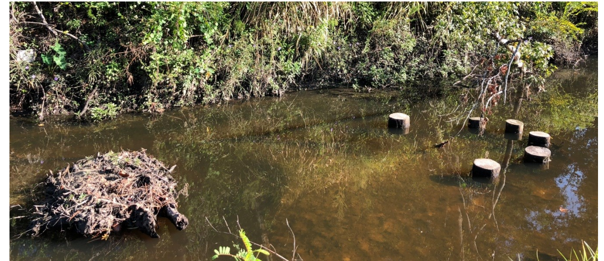
Boulder Habitat Cluster. Array of stumps and logs driven into the streambed at prescribed spacings to create refuge for small fish species and turtles.
