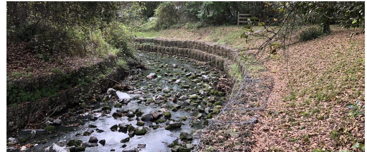
Gabion baskets along Lake Parker Canal, Polk County Florida.
